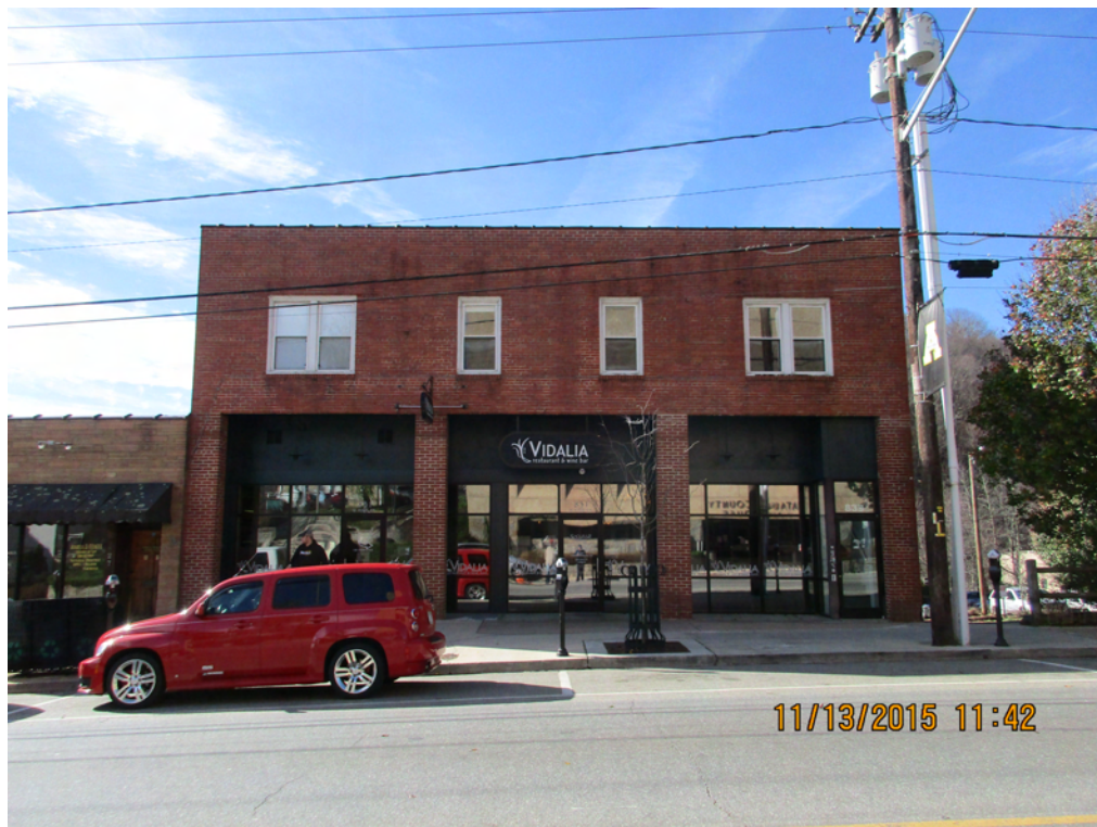
The Edmisten Building (WT0883) as it appeared in November 2015. Image by Eric Plaag.
