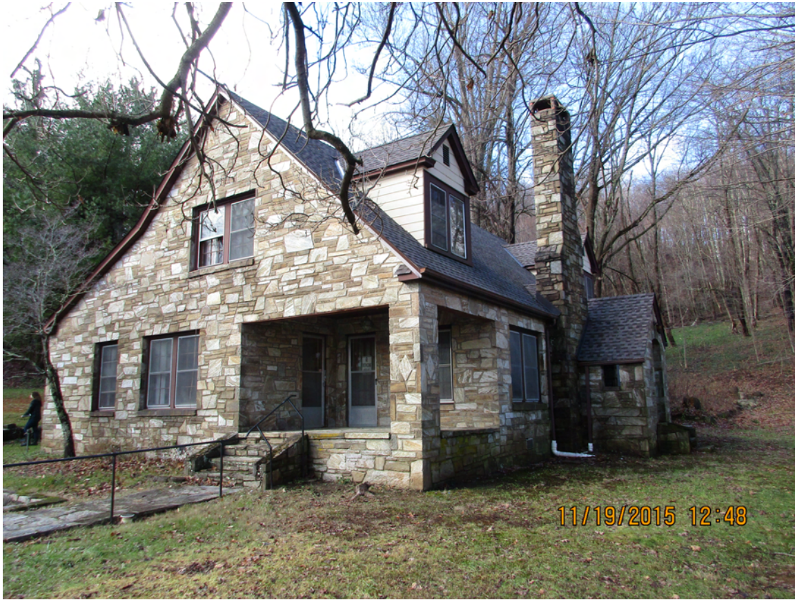
The R. L. Clay House (WT0530) as it appeared in November 2015. Image by Eric Plaag.
