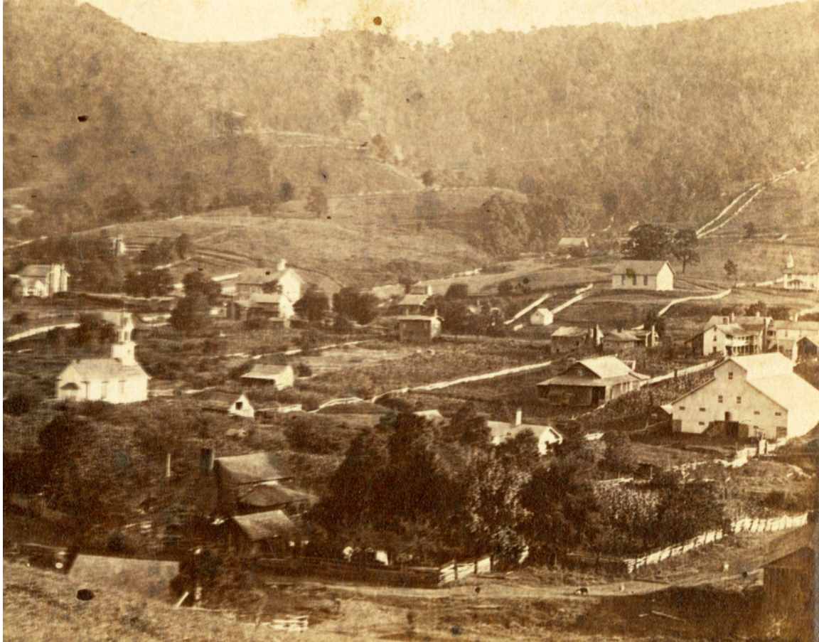
Boone as it appeared about 1885, looking toward the northwest from a point just south of present-day Depot Street. At far left is the first Boone Baptist Church, with the 1875 Watauga County Courthouse located at center left. At far right is the Critcher Barn with the W. L. Bryan residence and the Blair Hotel located just north of that. Image by L. A. Ramsour, courtesy of the Historic Boone Collection, Digital Watauga Project.
