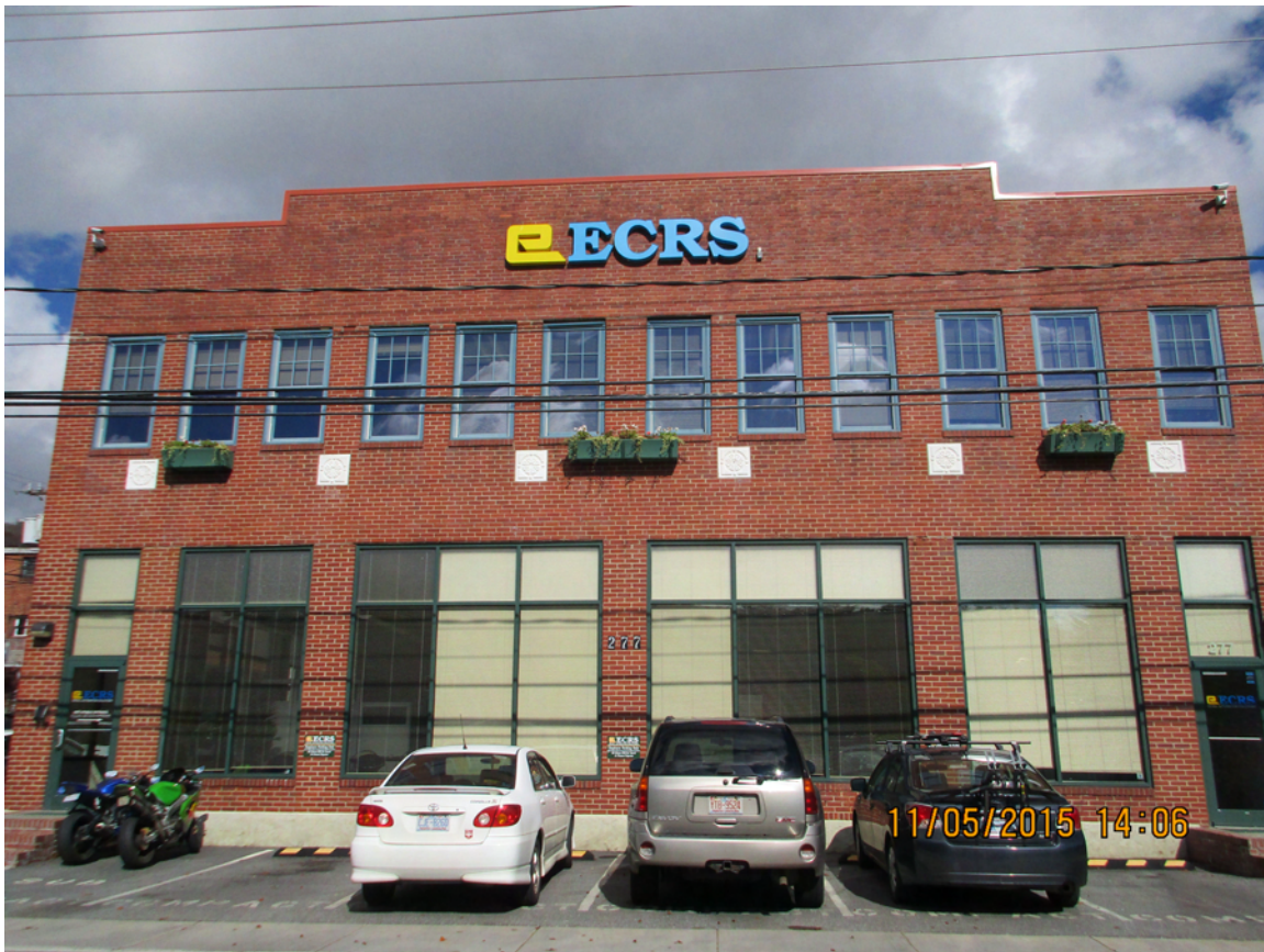
Winkler Motor Company Building #1 (WT0600) as it appeared in November 2015. Image by Nicole Holladay.
