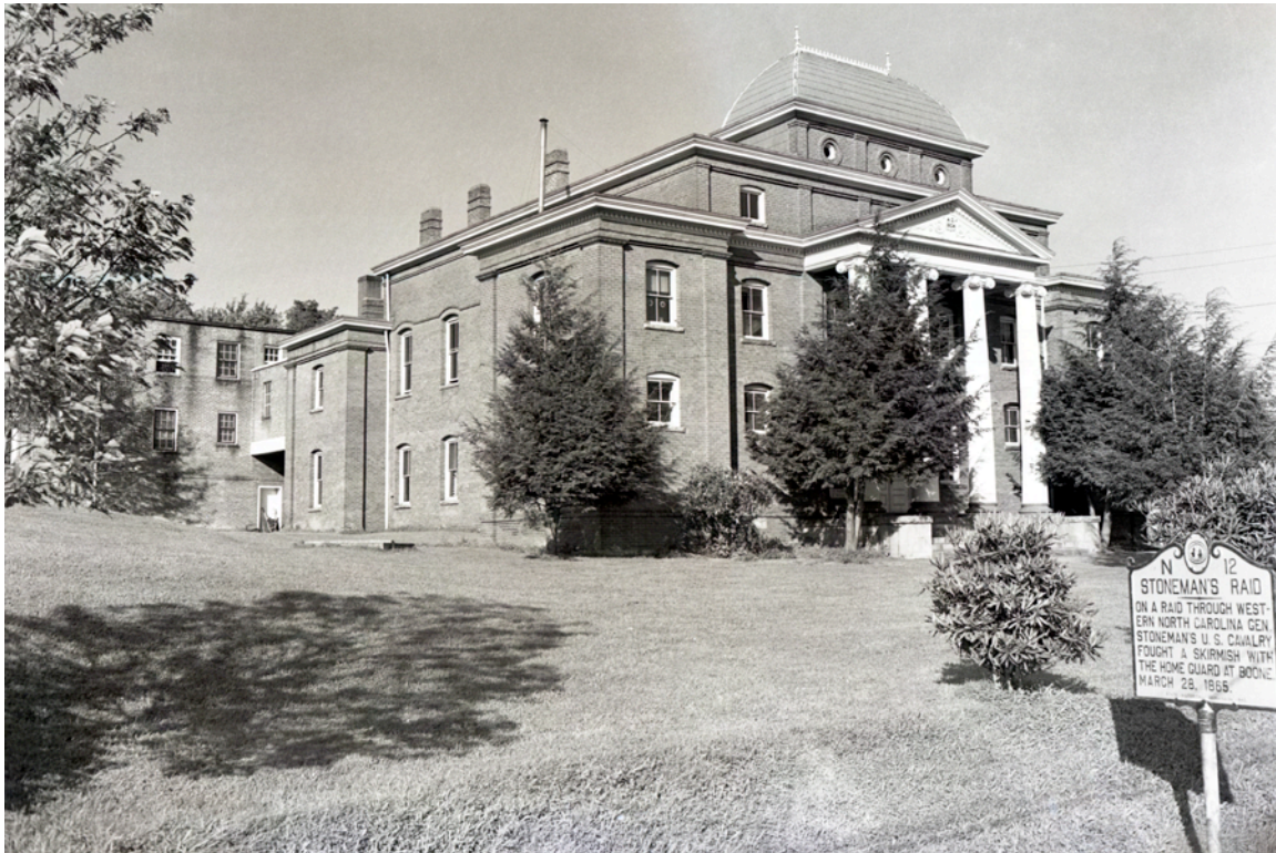
The 1905 Watauga County Courthouse (with the 1927 jail at rear) as they appeared in the 1950s. Image courtesy of the Palmer Blair Collection, Digital Watauga Project.
