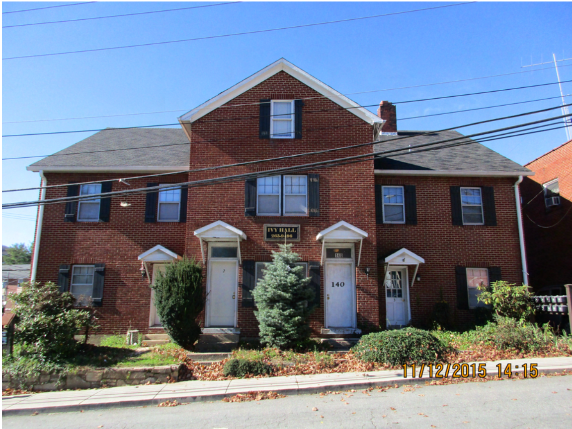
The Dr. H. B. Perry Building (WT0844) as it appeared in November 2015. Image by Eric Plaag.
